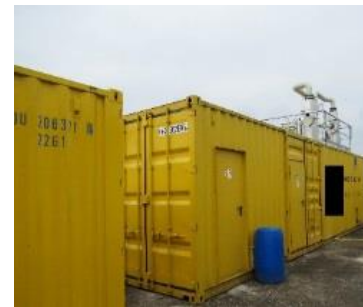
Photo 1: air scrubber (left) and ammonia stripping / scrubbing installation (right) (© VCM)
