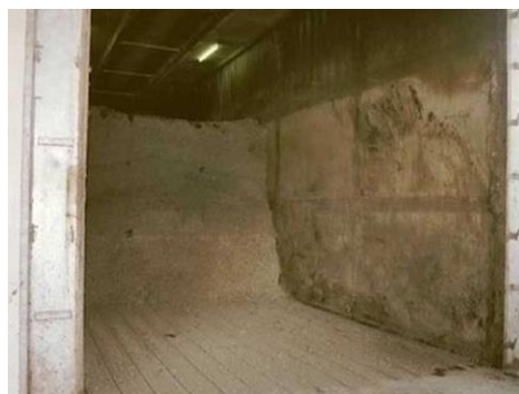
Figure 2-24 Biothermal drying. Source: VCM
