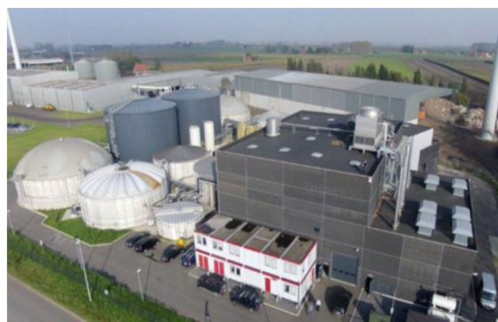
Figure 1. Aerial photo of the demonstration plant Waterleau NewEnergy.
