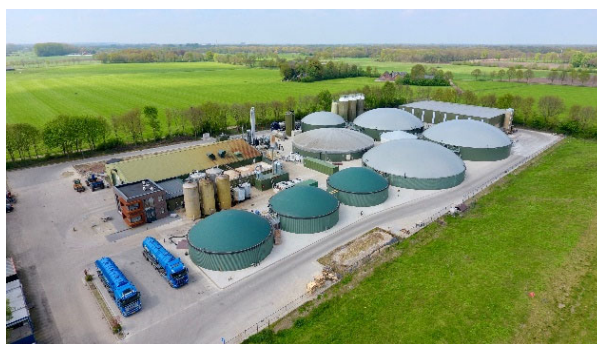
Figure 1. Aerial photo of the demonstration plant Groot Zevert Vergisting.
